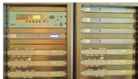
A Dante digital network has been created with the addition of BSS Audio BLU326 and BLU-B0B processors
