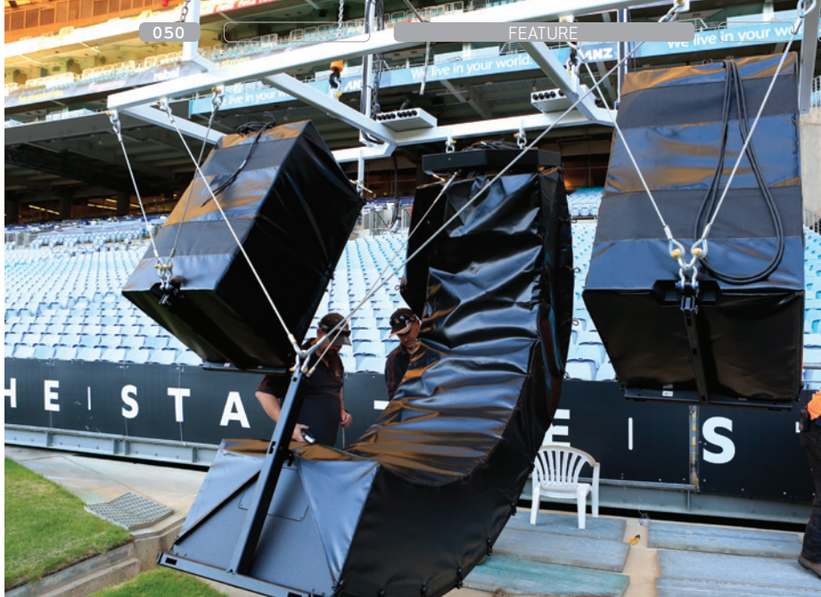
Top: One of the arrays comprising a line of 12 d&b Vi8 elements and a vertical pair of Vi-Subs either side along with the custom steelwork and rigging designed and built by the PA People. Precise geometry and calculation of each of the speaker cluster and frame elements was required in order to maintain the balance of the cluster, with some clusters weighing almost a tonne and measuring almost 7m in length.
