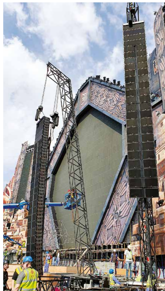
The main hangs each consisted of 20 K1s
