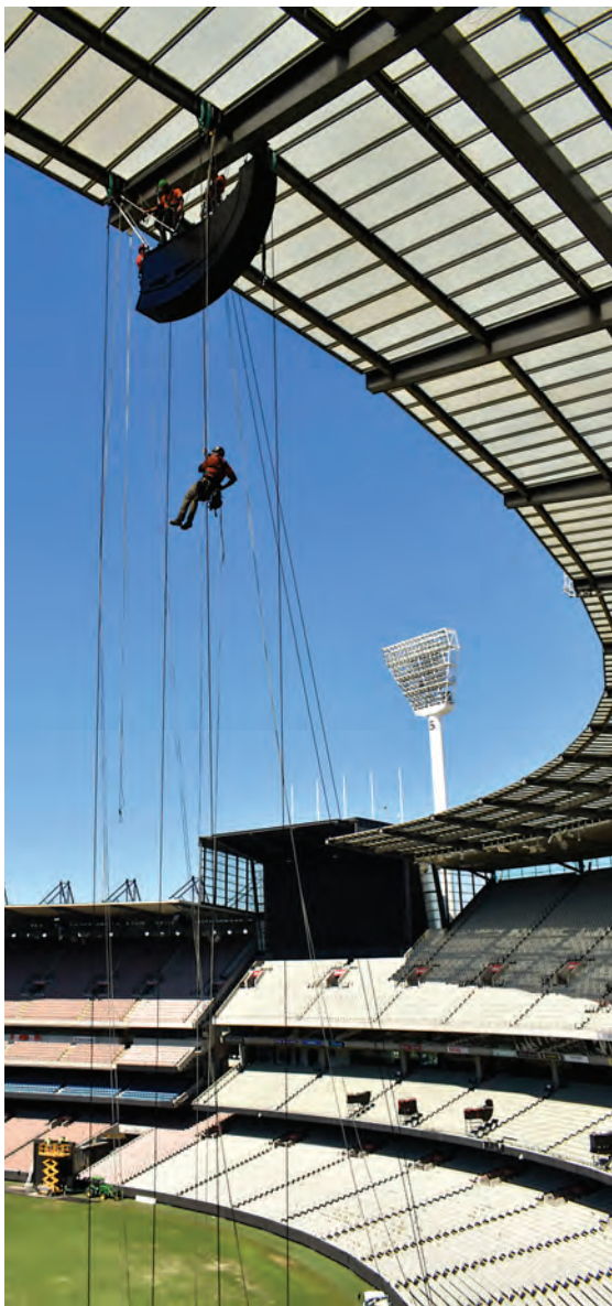
Technical riggers attach arrays at 40m up
