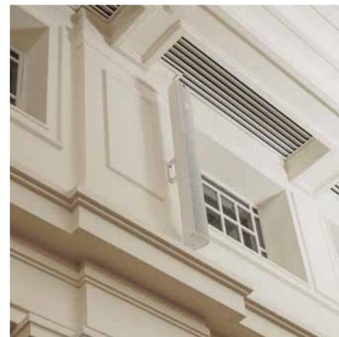
the audio routing in the installation. The correct speaker pair for each orientation is selected using a Crestron control system, accessed by a discreet wall-mounted touch panel or an iPad running Crestron's XPanel software.
